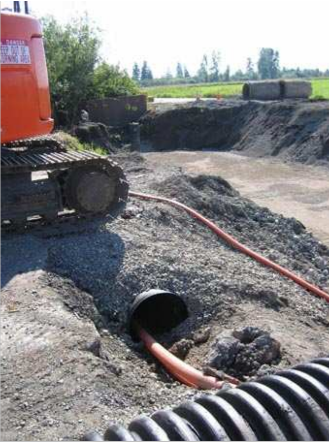
Here is a Qwest cable being rerouted for the ghost fish
